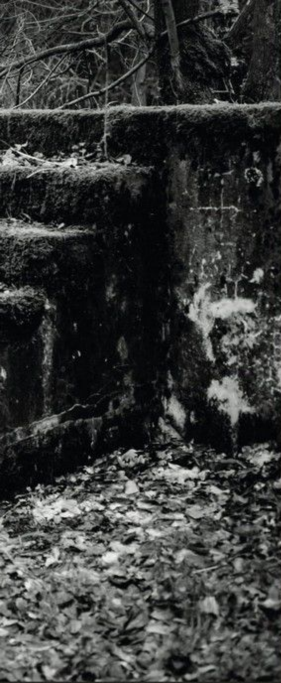
Fragment of the swimming pool from the 1930s in the area of Stalag VIII B (344) Lamsdorf
